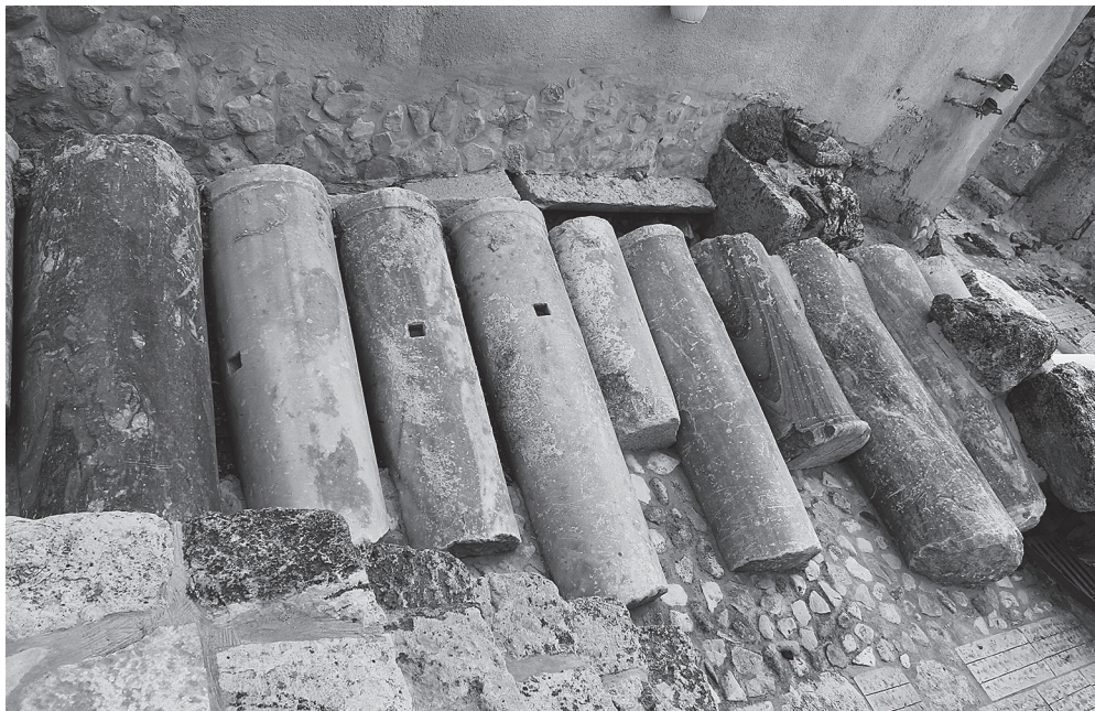
Il.9. Complete monolith column shaft, carved from Carystian marble near the Tomb of St. John inside the Latin Cathedral. Photo credit: S. Tarkhanova (2019)
