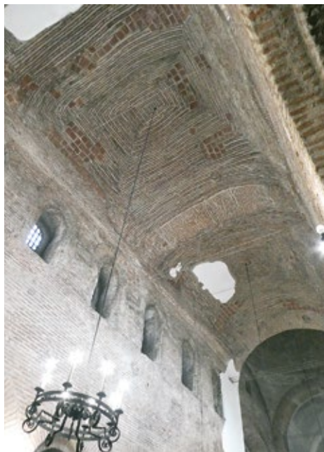
Fig. 5. Sofia, Saint Sofia. Vaults of the nave
