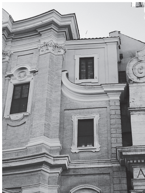
10. Francesco Borromini: Oratorio dei Filippini, detail of the transition between the façade and the existing church designed by Antonio Rughesi
